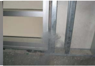
Air Leakage
