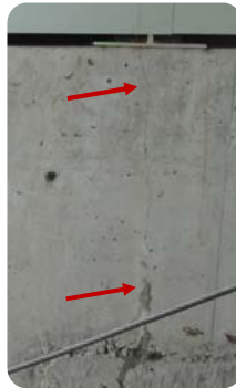
Concrete cracks
