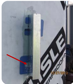
Z-girt fasteners
