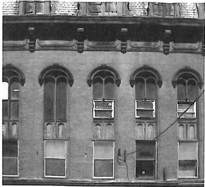
The damage wrought by replacement windows is self-evident and increasingly pervasive. All photos: © Walter Sedovic Architects
