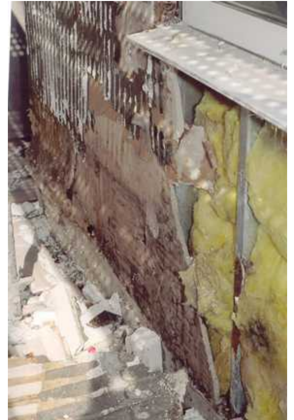
Rot & Corrosion
